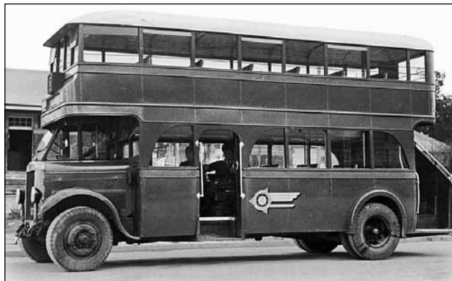
TD1 No.11 showing its front entrance and strengthened body
