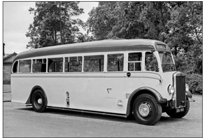
The Tiger TS8, DDG 900, with new design of Leyland body, sold to Cottrell, Mitcheldean (BVCMT L024011)
