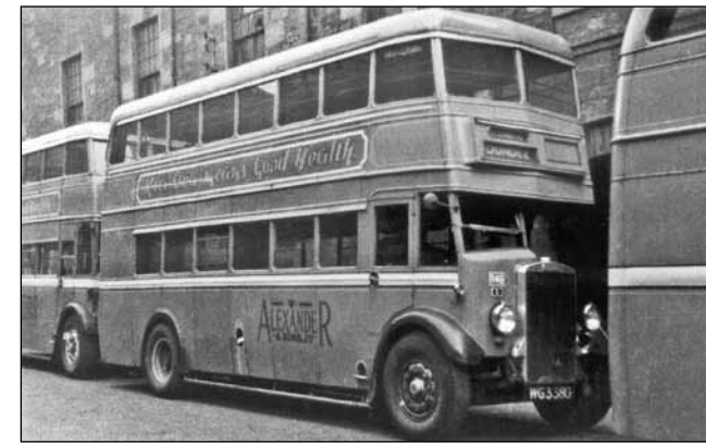
R46, WG 3380, in Dundee showing the initial rebuilding evident with the wide pillar behind the cab door.
