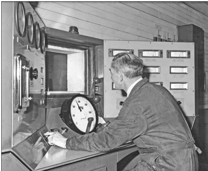
View of one of the L60 development test beds in the Research Department at Spurrier Works dating from the 1960s. The left-hand side of the console contained pressure gauges to monitor coolant and oil pressures and Leyland's own design of fuel meter, at that time fuel consumption would have been measured in lbs/h. The lever next to the testers left arm is connected hydraulically to the throttle lever on the fuel pump, the large white gauge in the centre displayed engine rpm. The gauges on the right-hand console are moving coil temperature gauges to monitor fluid and gas temperatures. Remarkably, even though a number of test beds in the Research Department were upgraded to computer control in the 1980s, this L60 test bed remained in this format right up to the department's closure in the mid 2000s and was used for testing reworked L60 engines for the Oman army.
