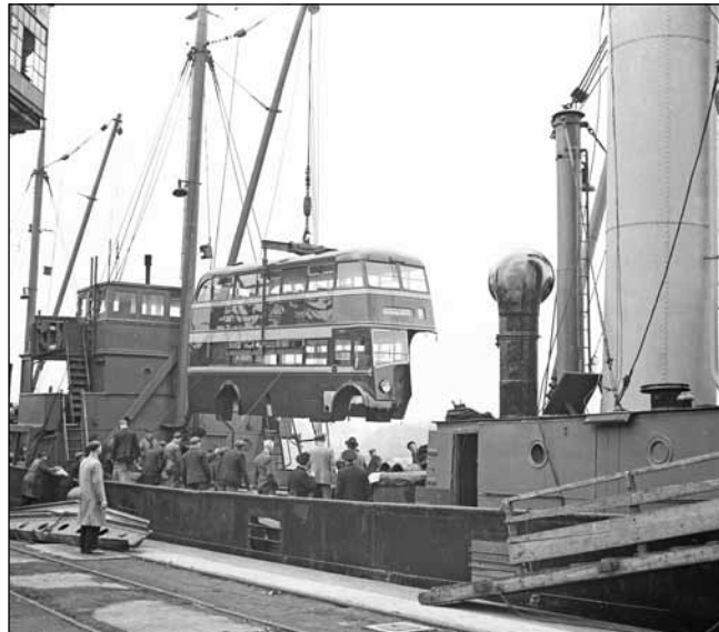
CIE took some of their deliveries as complete vehicles and others with chassis & body separate to minimise customs duties. Here a body is being loaded at Preston docks en route to Larne (BCVMT L034888)
