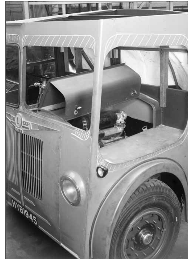
One of a series of mock-up full width cabs which were not proceeded with due to objections by the Ministry of Supply (BCVMT L027617)
