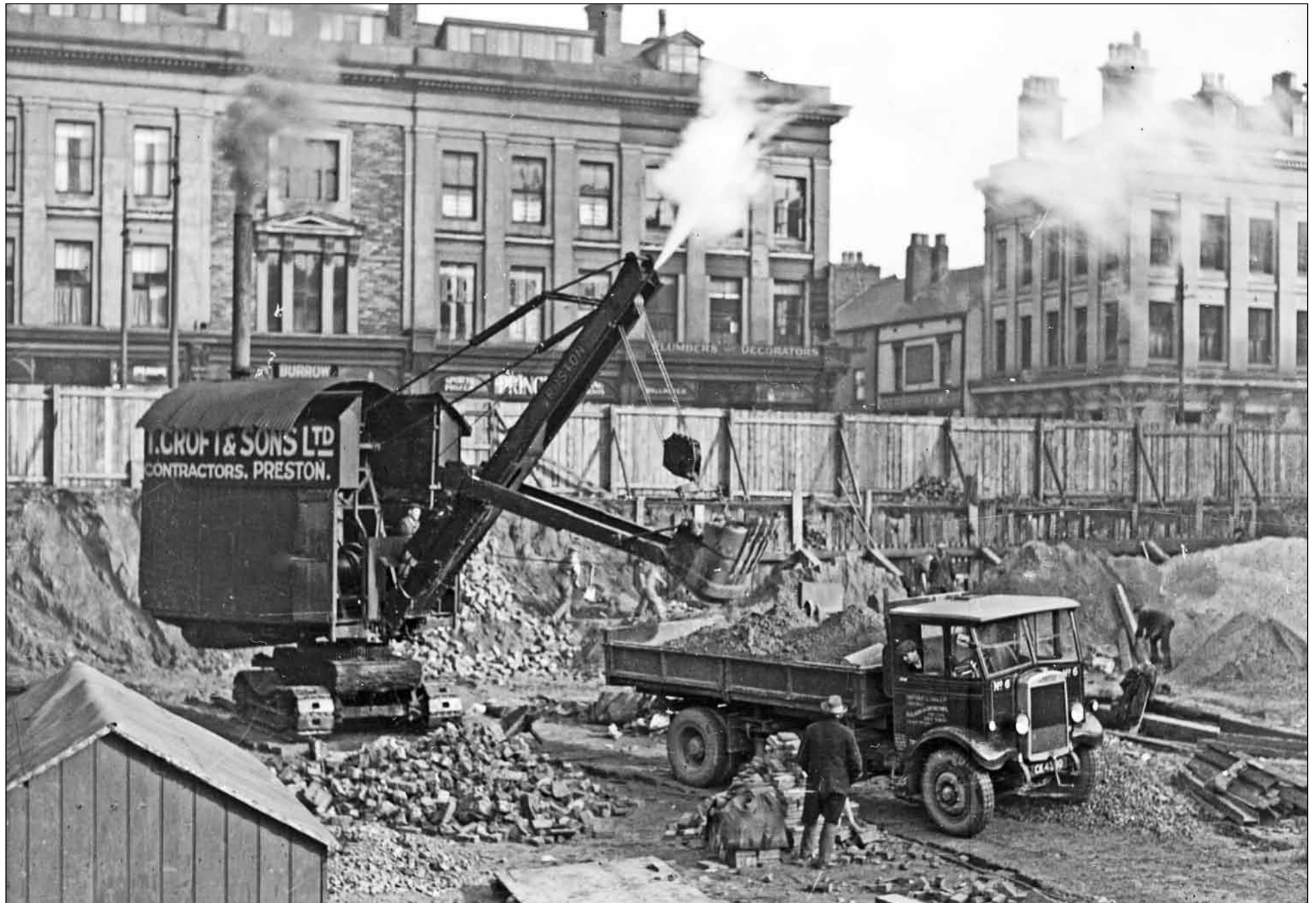
A Ruston steam shovel in its heyday, snorts fiercely as it loads one of Thomas Croft's two Leyland Bulls, CK 4390, a TSQ2 tipper (chassis 66510) in Preston in March 1931.
